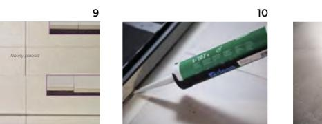
16 Edge joints occurring at corners, changes of paving level and changes of material should be covered with tile trim or a tile itself and sealed with flexible sealant. Minimum joint width: 8 mm.
