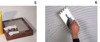
5 Choose the type of adhesive depending on the conditions used. The choice of tile and adhesive are critical to the subsequent performance of the entire work. Factors to take into account are: the type of ceramic material, tile format, substrate and end use (any traffic it will be subjected to, safety requirements in respect of falls...) PORCELANOSA catalogues contain recommendations in respect of use and slip resistance, as well as the butech adhesive recommended for each design.
