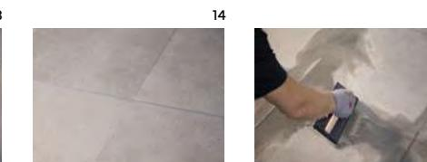
20 Joints should be grouted when the tiles are completely fixed to the substrate. In respect of paving, follow the recommendations of the adhesive manufacturer to ensure sufficient time is allowed before the floor is walked on or subjected to load. In this way movement and/or breakages are avoided.
