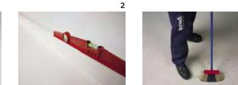
3 Surfaces to be tiled must be completely free of dust or any other substance which could impair tile adhesion. For specific installations (radiant heating systems, façades with mechanical anchors, ceramics on roofs/ceilings or particular design constraints) request additional information specifically for each application.
