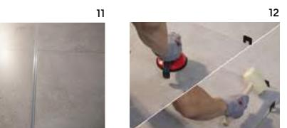
13 Great care should be taken when handling to avoid scratching, breaking or chipping the tiles, especially rectified tiles. Prior to installation, check that the tiles are free from defects.
